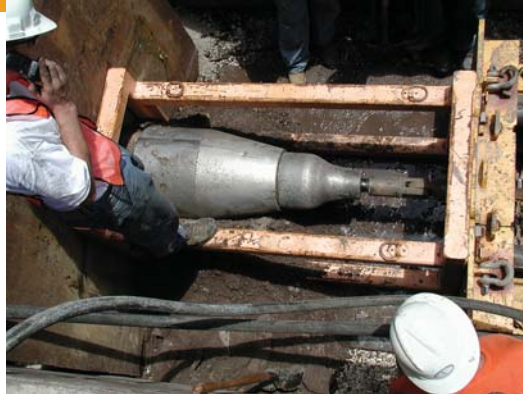
Far left: A pipe insertion pit. Left: The Air Impactor arrives.
